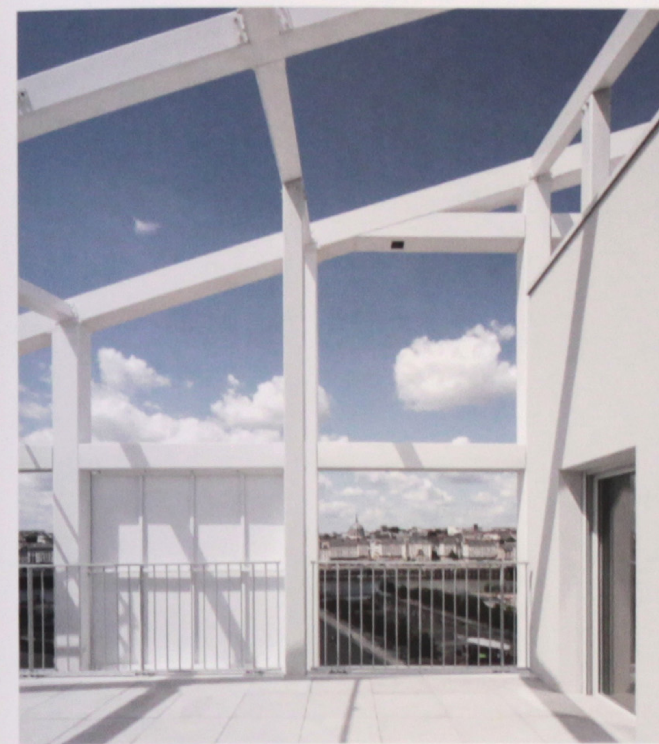
↑ Whether the facade grid is opened or screened depends on the function of the space behind it.
